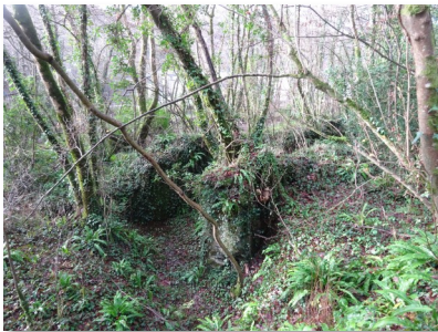
Lock 21 : Chamber and Downhill Gates mountings, 2018
