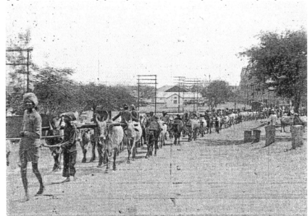
Cylinder for Winding Engine on way to Circular Shaft. Weight 15½ tons.
