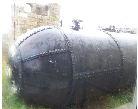
Cornish boiler, King Edward Mine.
