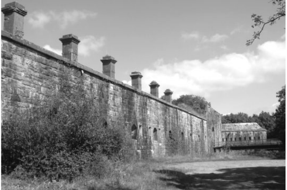
The wide area next to the imposing East wall of the fort, which was used as a railway marshalling area.
