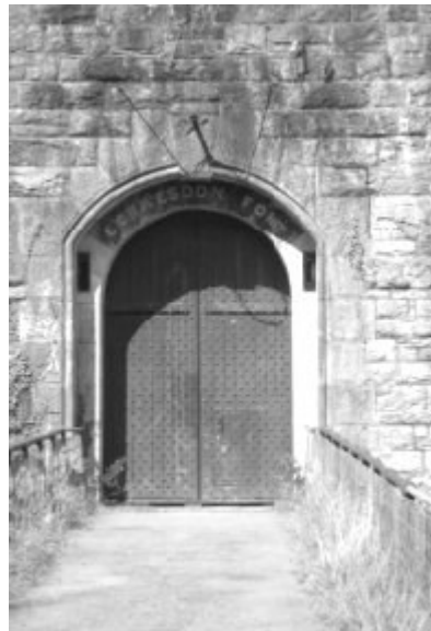
The imposing front entrance to Scraesdon Fort.
