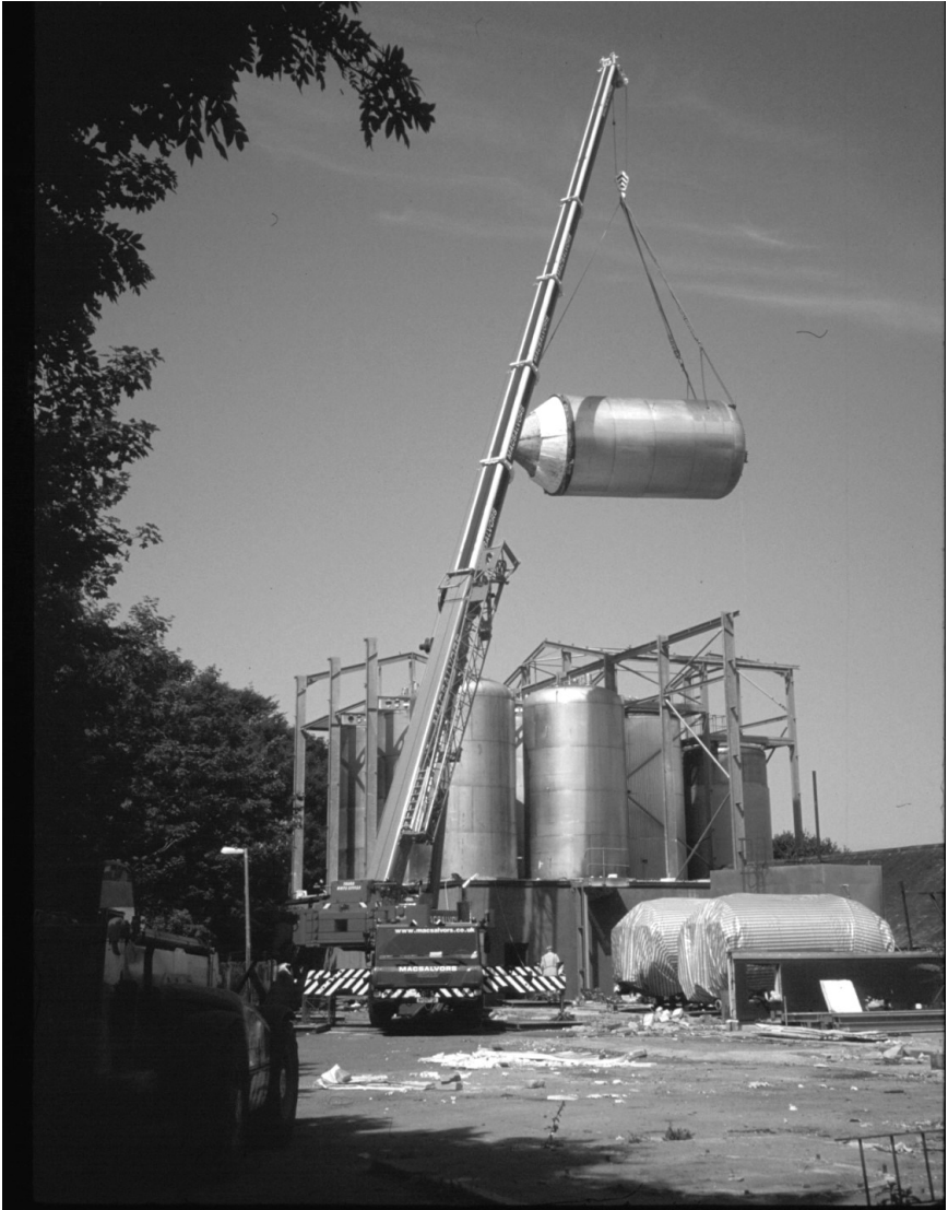
Macsalvors crane lifts out one of the giant storage tanks from Redruth Brewery.
