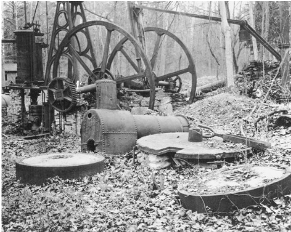
Figure 3: The Vaucluse beam engine in 1931, showing fragments of the Chilean mills and fallen balance bob.
