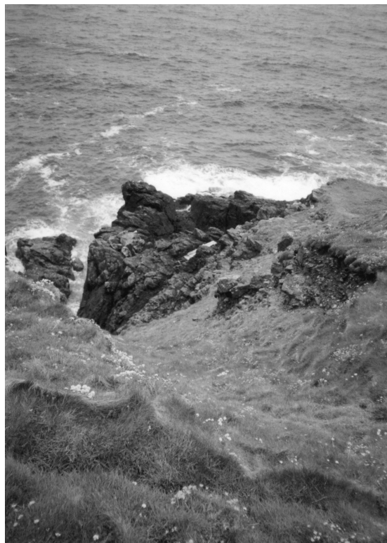
Wheal Unity, showing cutting down which the water balance was assumed to run, and (above centre) the boarded over shaft; whim plat to right.
