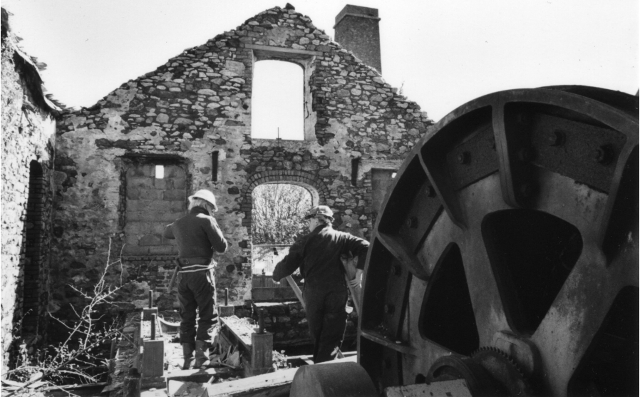
Cap'n Clive and Kingsley Rickard surveying the New Dolcoath winder
