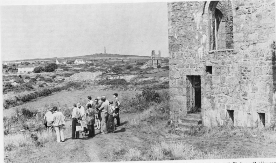
Society's Summer Weekend: Participants being entertained by Jack Trounson in the shadow of the Frazer & Chalmers Reidler compressor house, Marriott's Shaft, Basset Mines. Beyond can be seen the bob wall of Thomas' 60, West Basset, and in the far distance Carn Brea monument.
