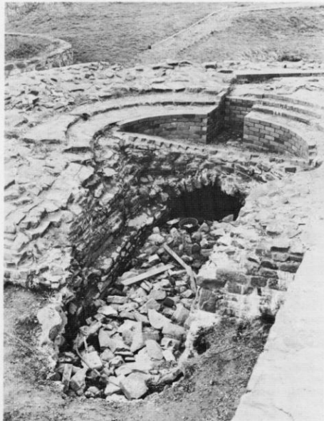
Haystack boiler excavation.
