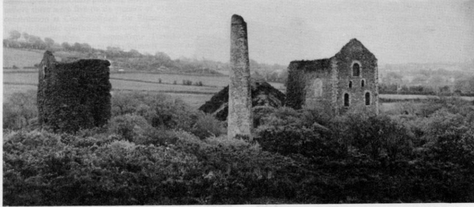
The pumping and whim engine houses and stack at Redmoor, near Callington, seen here in 1981, have been demolished in connection with SW Consolidated's bid to reopen the mine for tin. The pumping engine erected by Harvey & Co. for the short reworking in 1888 is believed to have been a 78-inch of upcountry origin.
