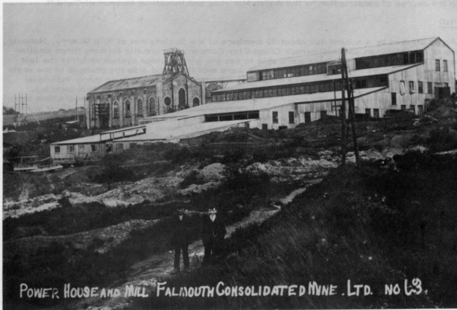
The power house and Mill at Falmouth Consolidated Mines Ltd. See the article on The Early History of Flotation. The photograph is from the collection of Mr. J. H. Trounson.
