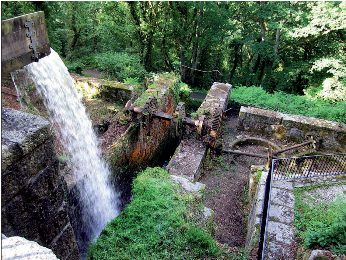
The well preserved rock grinding mill, fed by the Carmears Leat. Two pairs of grinding pans were worked by a central waterwheel, its axel balanced on the two walls.
