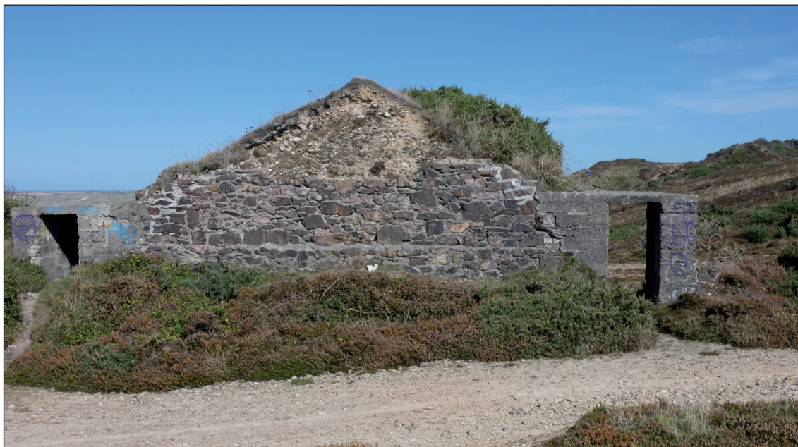
A very complicated feature! This is the south side of the protective mound which formerly ran around a possible mixing house. The masonry is one of the tramway tunnels which leads up to the cartridging huts. During World War 2 the feature was extended north and south with concrete blocks to form air-raid shelter.
