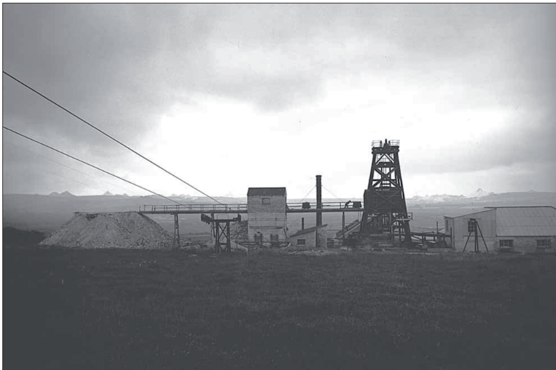
New Shaft, at the southern end of the workings, on the southern slopes of Castle-an-Dinas hill. The horizontal beam on the right of the headgear operates the pump and the hoisting engine house is behind the headgear. Trucks from the shaft cages are run along the gantry to dump waste rock on the left, and the ore is tipped into the ore-bin (centre) from which it is conveyed to the mill at North Shaft by overhead ropeway.
