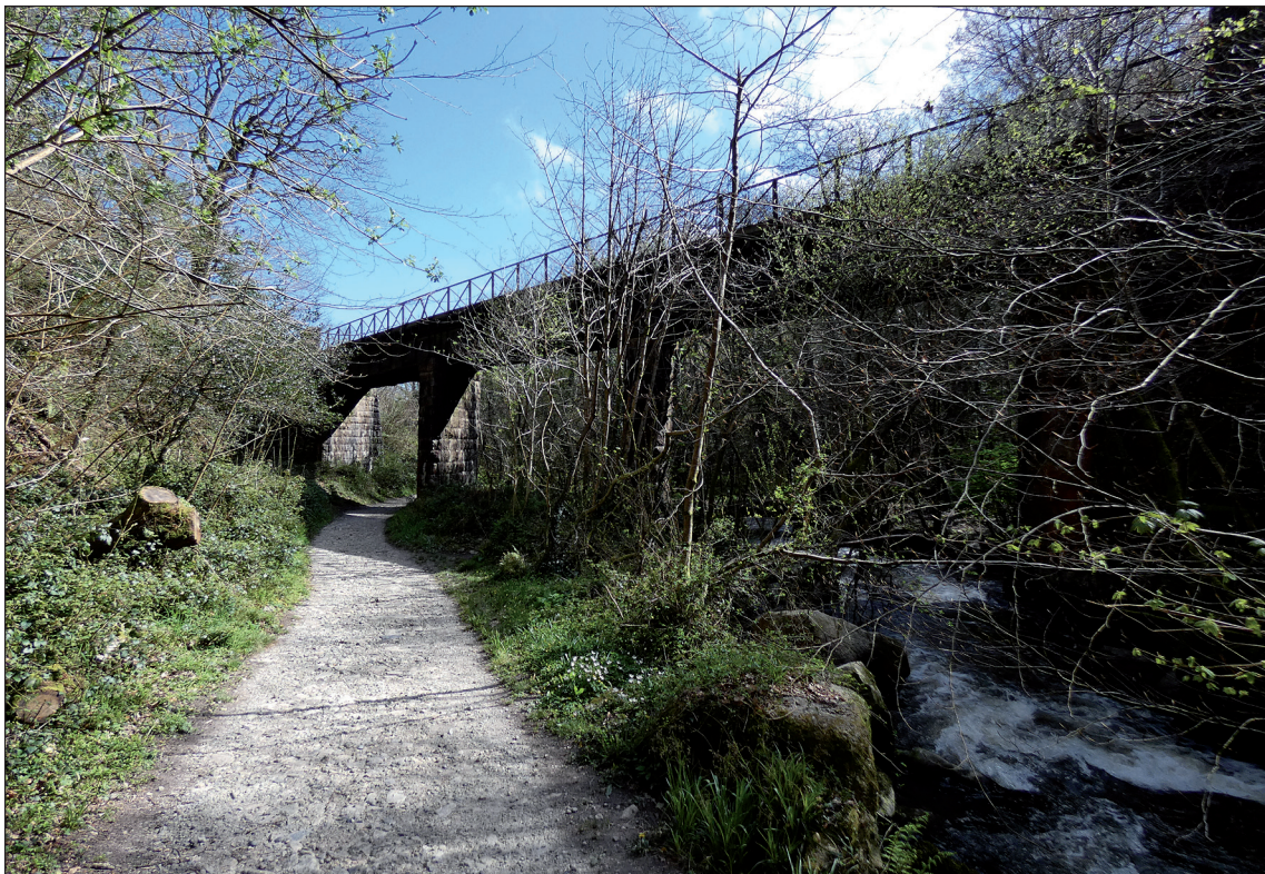
Modern railway bridge carrying the Newquay-Par branch line over the Par River and the lower tramway. Granite tramway sets can be seen in the former trackway here.
