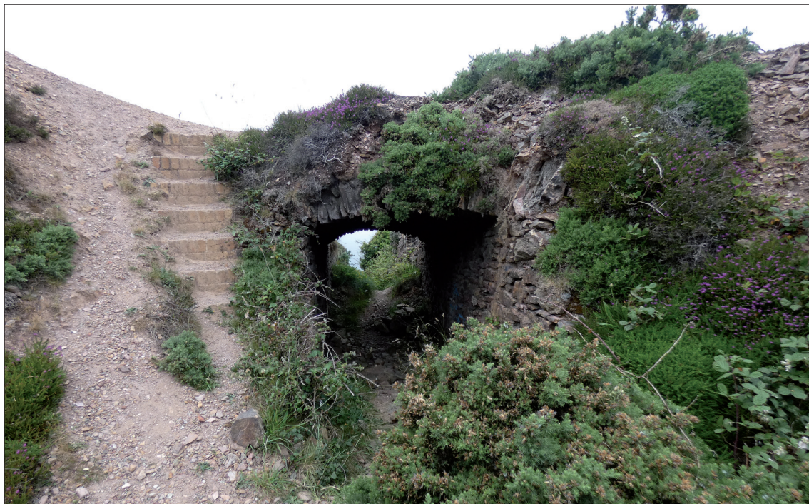
Nitroglycerine tunnel leading from A2 nitrating house to B2 separating house. The tunnel now terminates in a very steep slope as the material of the cliff slope, as well as the protective mound for B2, was removed for hard-core in the 1960s.
