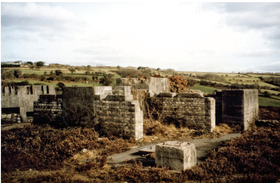
Terminus of the overhead ropeway from Park an Chy; the Nissen stamps loadings are on the left.
