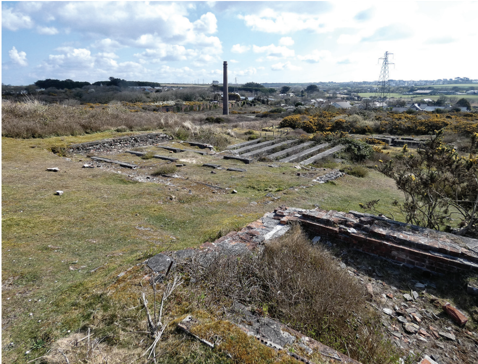
Part of the service area: possible small magazine in the foreground and filter room with associated water tank loadings in centre. Beyond that are concrete loadings for heavy machinery. The nitric acid factory and the remaining stack are in the background.
