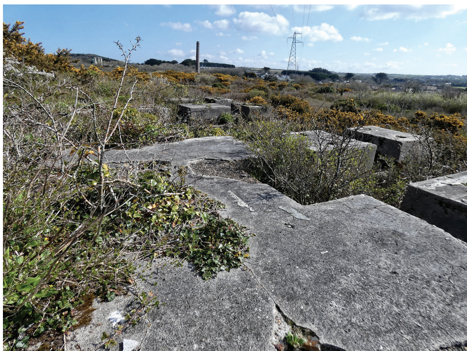
House for two Holman Brothers twin horizontal engines, used for operating the pumps in Boiling Well Engine Shaft.
