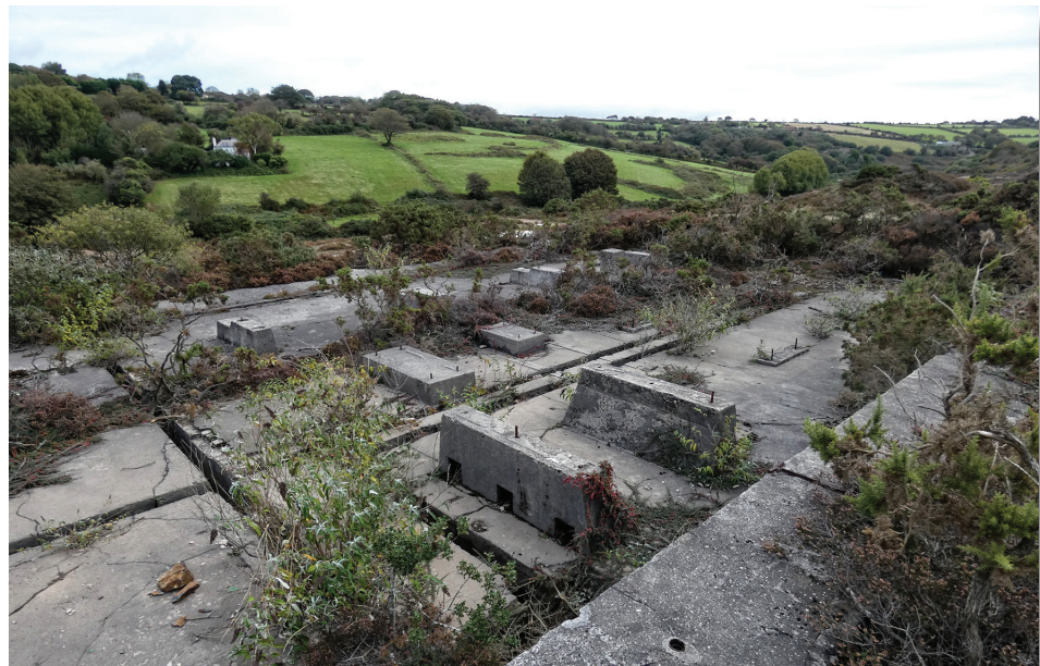
Looking down on the 20th century mill showing the typical cement-faced concrete floors and loadings. Gutters run parallel and across the floor. The stamps loadings are just to the right of the photo.
