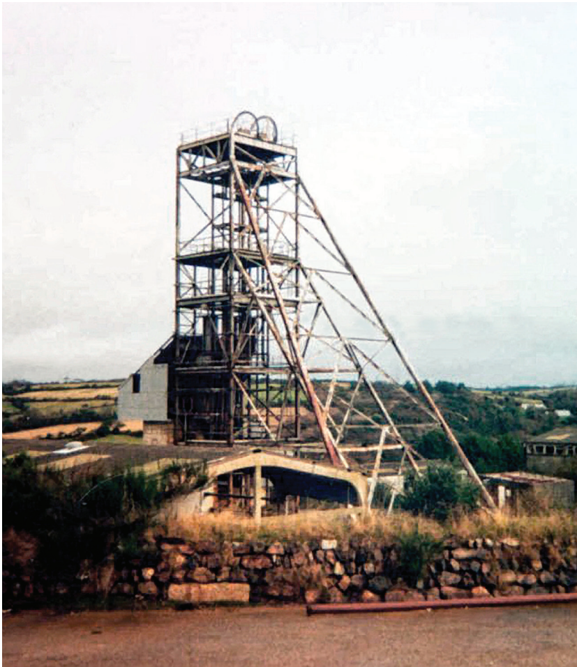
The well-known haedframe over the engine shaft at Mount Wellington.
