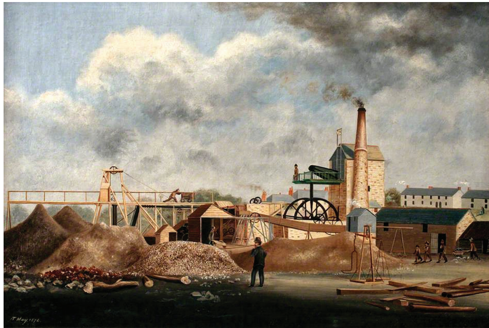
A marvellous picture of the Restronguet Creek Tin Stream Company's works to the south-west of Point. Piles of sand, presumably waste, can be seen around the works; the stamps can be seen to the left of the engine house, with a long gantry where a man is pushing a small wagon of ore towards the stamps. Painting by T. May, 1874, at the Royal Cornwall Museum.
