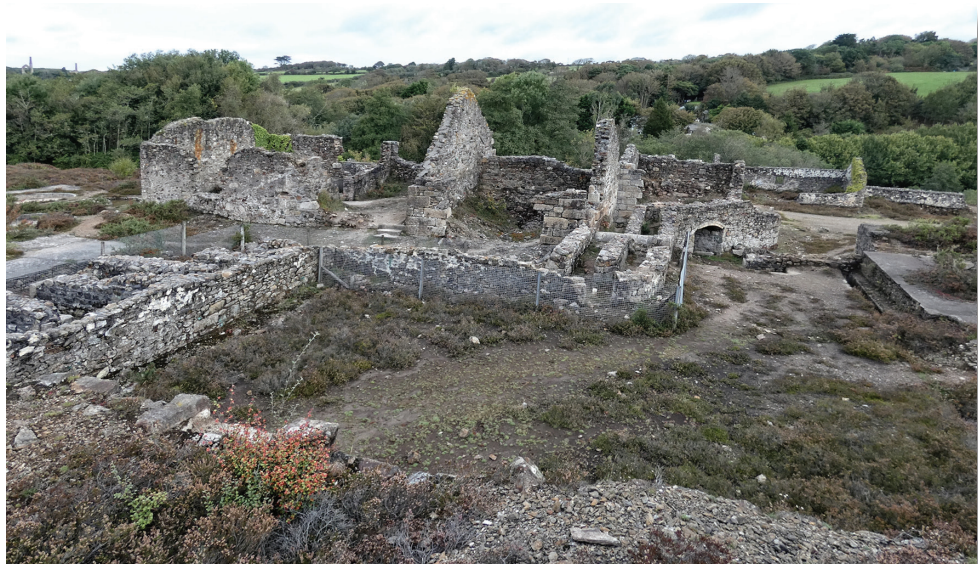
The Poldice arsenic works: Brunton calciners on the right, mills centre and first labyrinth on the left. The 20th century mill is just to the right
