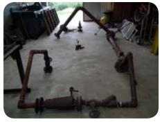
into water. Due to the lack of drainage in several places, a large quantity of standing condensate was causing water hammer and corrosion in the pipe. Finally, following comments by both the Boiler Engineer and the Inspector that the design would encourage pulsing, the decision was taken by the National Trust to replace the pipe work during the winter maintenance of 2018/19.
