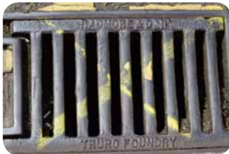
The drain cover in Truro.
