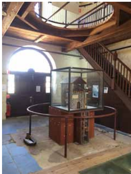
Fig. 10: Lower chamber (with cylinder bedstones) and middle chamber floor of the refurbished house of Morphett's pumping engine at Burra Mine with a working model occupying the cylinder position.
