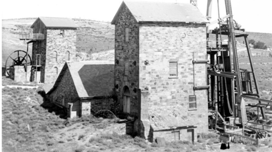
Fig. 9: Morphett's 80-inch pumping engine and 20-inch whim (and their shared boiler house) at Burra Mine in ca. 1904. Johnny Green, the Burra miners' mascot on top of the shears now stands atop the repositioned stack of Peacock's engine at the entrance to the mine site (State Library of South Australia, photo PRG 733/507)
