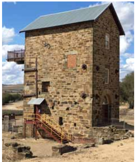
Fig. 8: House of Morphett's 80-inch pumping engine at Burra Mine showing the boiler house door, steam inlet and drain. In the foreground is the base of the boiler house.
