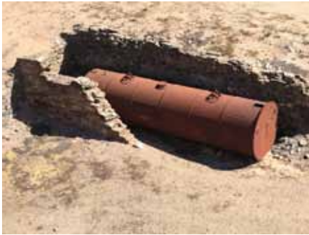
Fig. 11: Cornish boiler in the extension to the boiler house of Morphett's pumping engine at Burra Mine added when Morphett's whim was erected in 1861.
