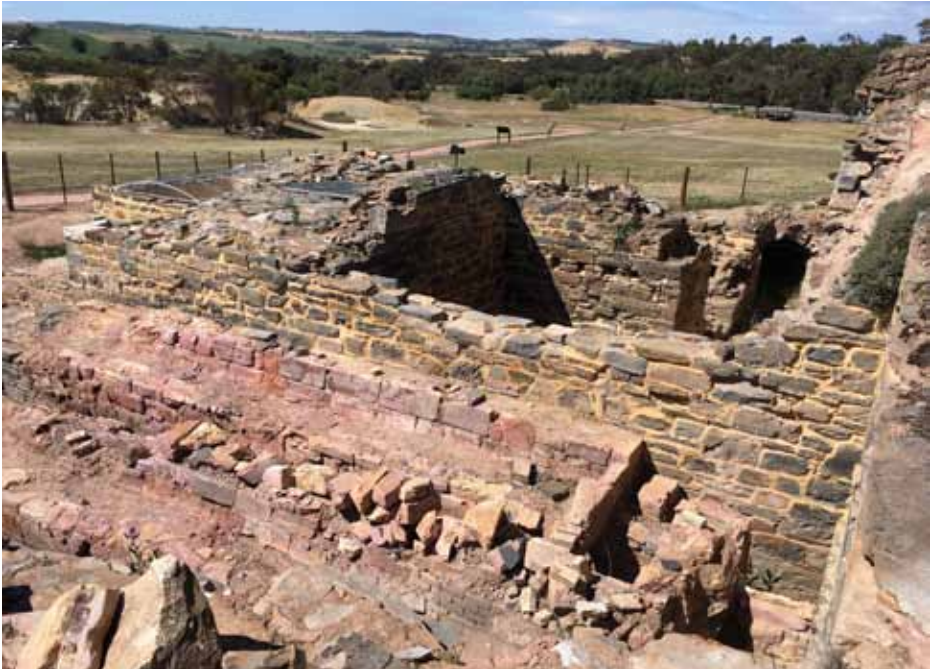
Fig. 5: Excavated base of the all-enclosed, 30-inch winding engine at Kapunda Mine showing the house of its two boilers (foreground), crusher house (right), and cylinder platform of the engine house (left) with its interior condenser pit covered by a flat grating.
